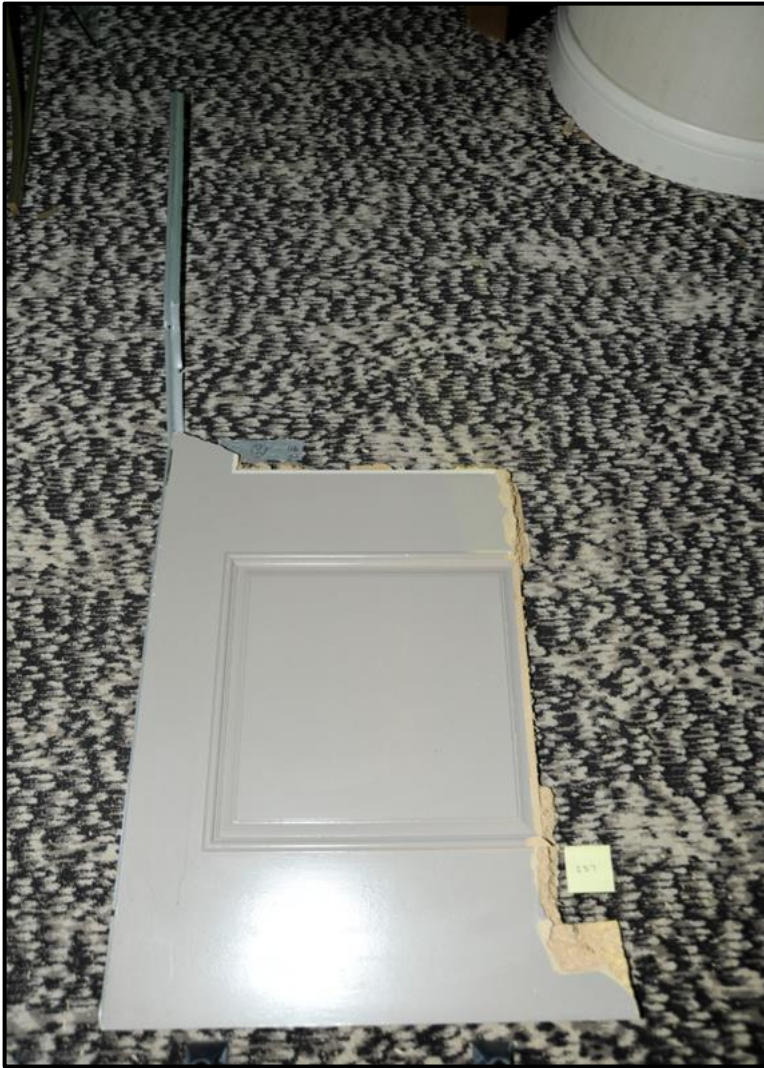
(Damage to entry door of room 32-135)
